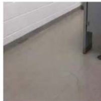
AES Replace Epoxy bathroom floors
