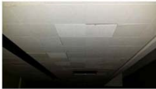
SMS Replace ceiling tile and ACM abatement (SMS)
