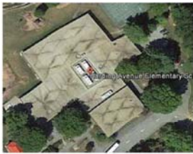
HAE HVAC Units Replacement
