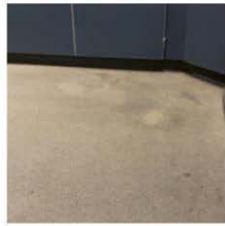
EMHS Replace Main office flooring
