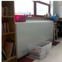
BEL Replace through-wall heating units
