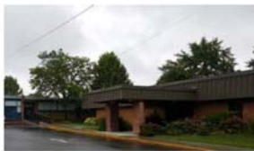
MBE Construct canopy from school to kindergarten
