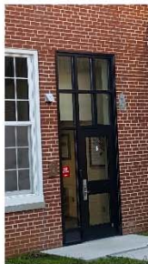
SMS, BHS Install canopy at main entrance
