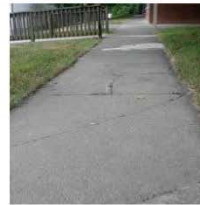
CES Replace deteriorated sidewalks
