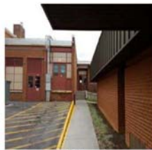
GLE Construct canopy over walkway between school and Kindergarten
