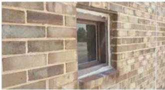
CHS Replace Library Windows CT
