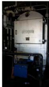
CPS Install new boiler - CT
