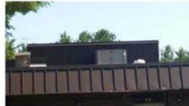
CPS HVAC Unit replacements
