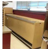
SMS Replace through-wall heating units
