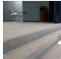
KES Replace Stage Flooring
